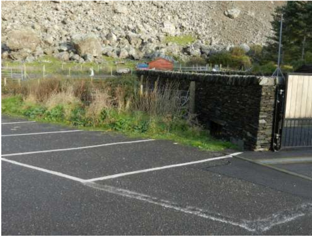
Appendix C – The boundary wall Seafari fuel store
