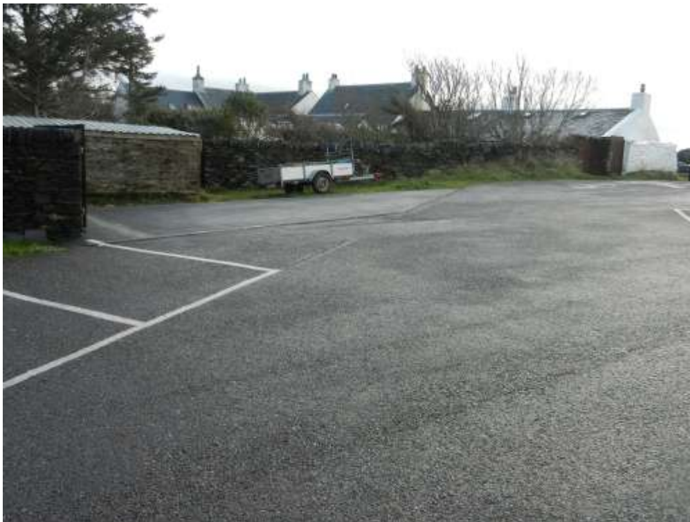
View from inside the car park back towards car park entrance
